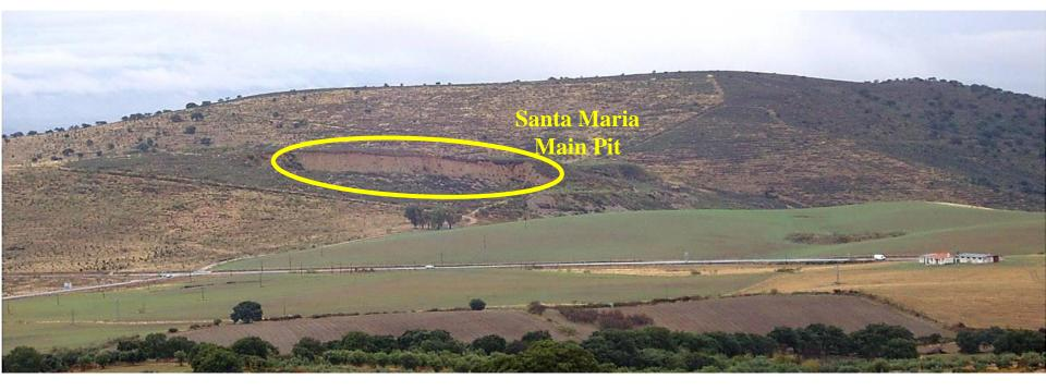
The small Santa Maria Mine, circled above, treated a colluvial tin deposit in the 1970s and 1980s. Unconfirmed official reports indicate a total historic production of 280 tonnes of tin from 400 tonnes of concentrate.
